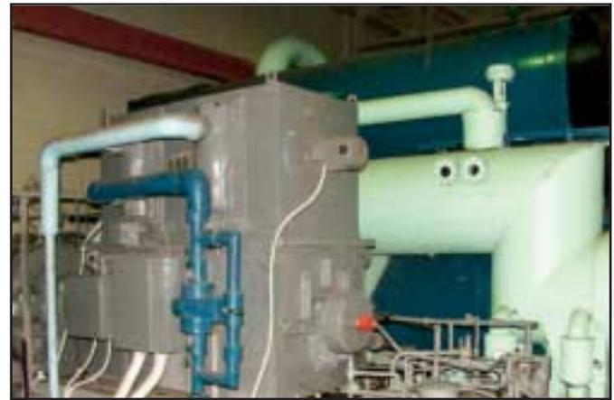
**Main chiller plant: 1969 vintage 2000-ton machine slated for replacement**
