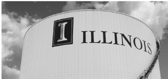
Chilled water storage tank
