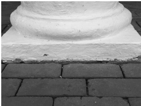
UNIVERSITY OF VIRGINIA Tuscan stone base before removal of patching and coatings
