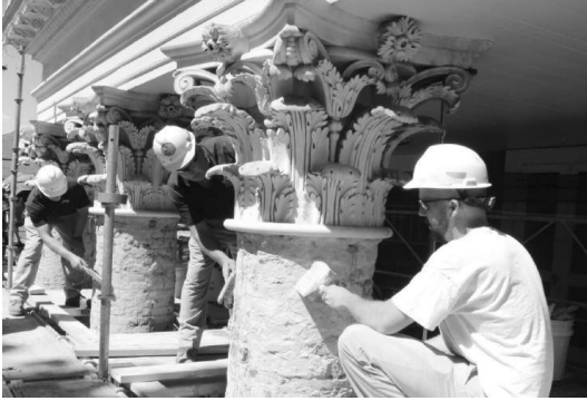
PAVILION III columns
