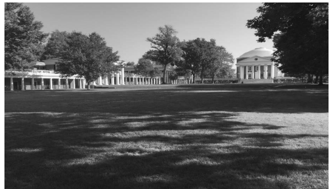
Fall of 2016 a project to restore the original Jefferson Tuscan columns was developed
