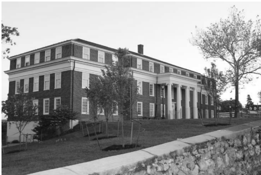
O'NEIL HALL newly renovated
