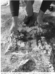
Falling roof at Glover - peeling membrane
