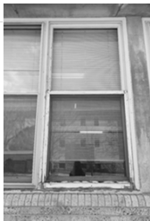
Failing single pane, wood windows in Shepardson
