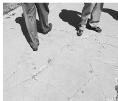
Cracked, failed sidewalks at Moby
