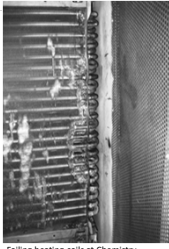
Falling heating coils at Chemistry
