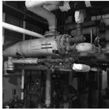
Old, inefficient heat exchanger
