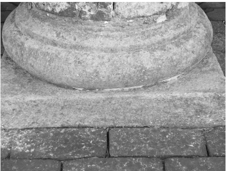
UNIVERSITY OF VIRGINIA Tuscan sand stone base after removal of coating and modern paints. Local sandstone was used to carve the original bases.
