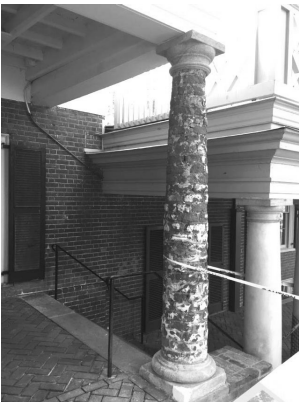
UNIVERSITY OF VIRGINIA Original brick column – cement plaster has been completely removed
