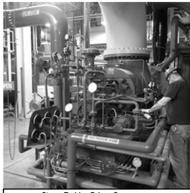
Steam Turbine Driven Compressor
