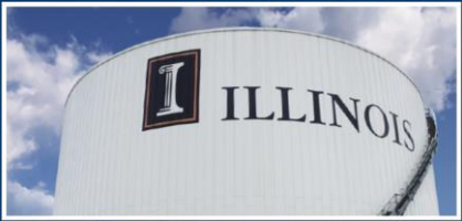
Chilled water storage tank
