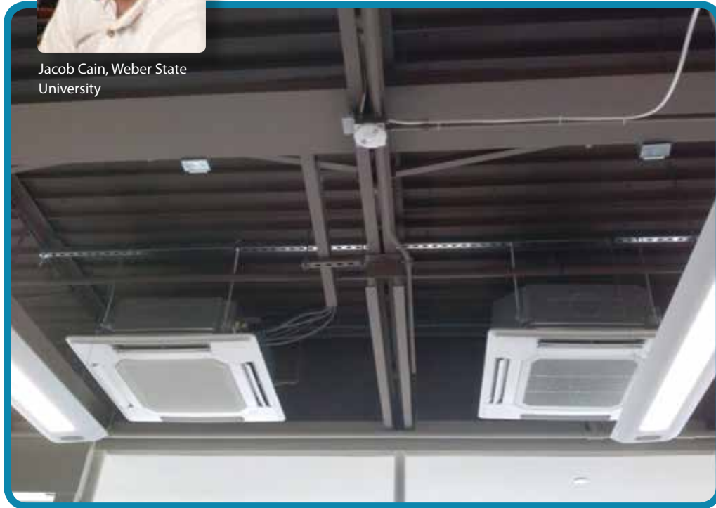
Terminal units in an office area running on water-cooled VRF at Weber State.
