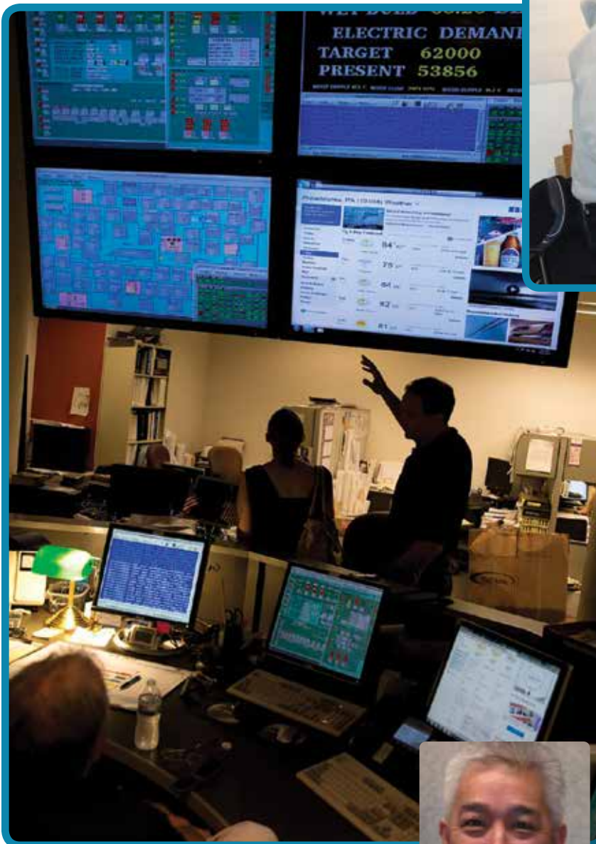
The University of Pennsylvania's Operations Command Center where staff manages campus facilities with the aid of an advanced Supervisory Control and Data Acquisition (SCADA) system that receives approximately 280,000 data points of information.
