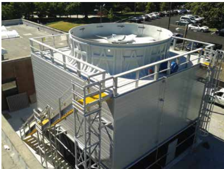
Tower – A new 3,000T field erected, FRP, counterflow tower includes low sound fan, double wall panel construction, access stair, and lightweight basin screens. The tower is designed at 80F wet-bulb and 85-100F temperature split.
