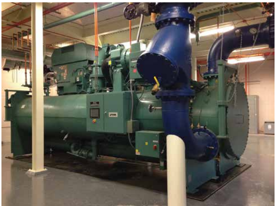
Chiller—GT's first medium voltage VFD chiller is a highly efficient 3,000T York YK-EP, R-134a machine. It was slotted into a bay originally designed for a 2,000T chiller.
