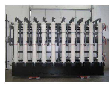
Graywater reuse solutions have used a combination of: filtration, microfiltration, ultrafiltration (shown above), and reverse osmosis.
