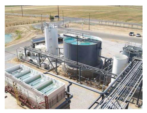
Cold Lime Softening Clarifier at a Western dry grind ethanol facility where a ZLD system was implemented. CLS is this decade's old technology that is making a comeback as it is common in
