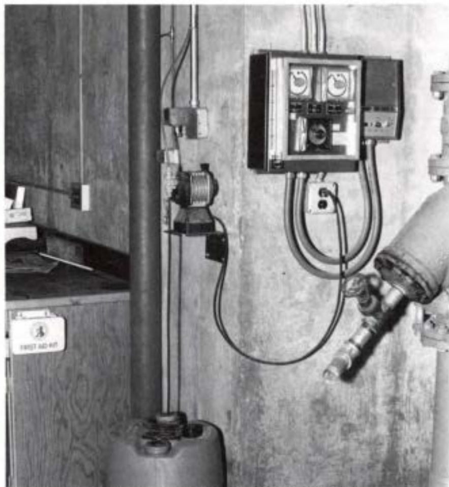
Conductivity monitor for "open" cooling tower. Monitor is located in basement mechanical room of three-story communications building.
