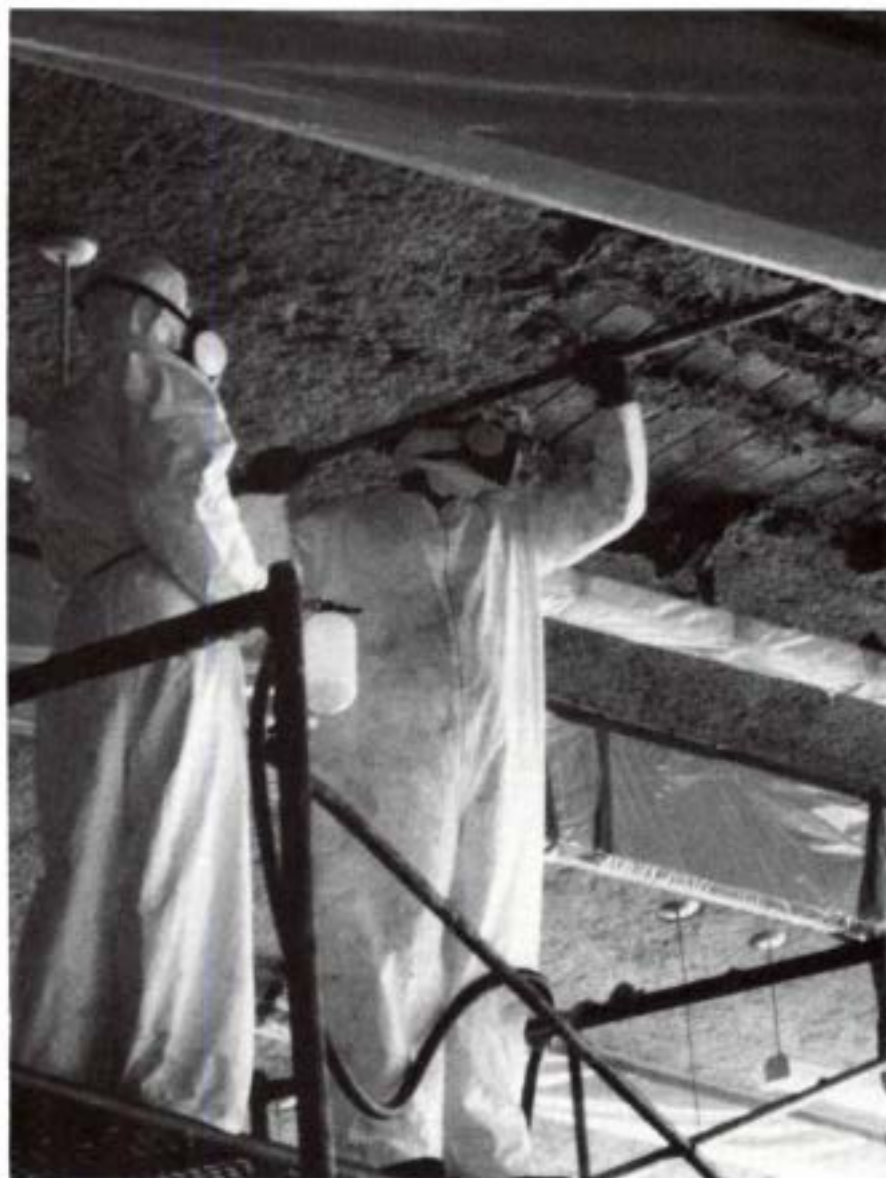
Workers removing asbestos from ceiling.
