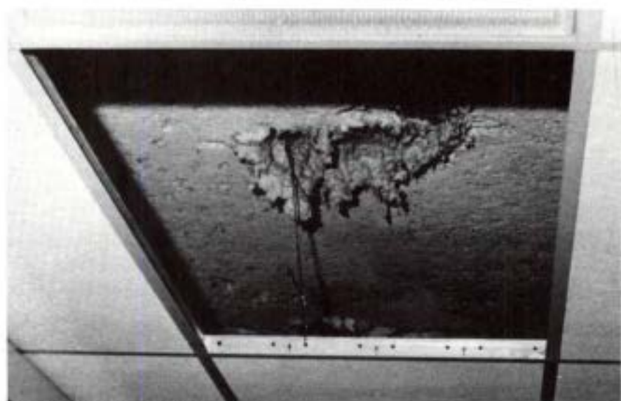
Friable asbestos above false ceiling.
