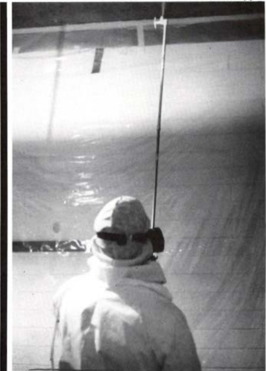
Worker spraying penetrating sealer.
