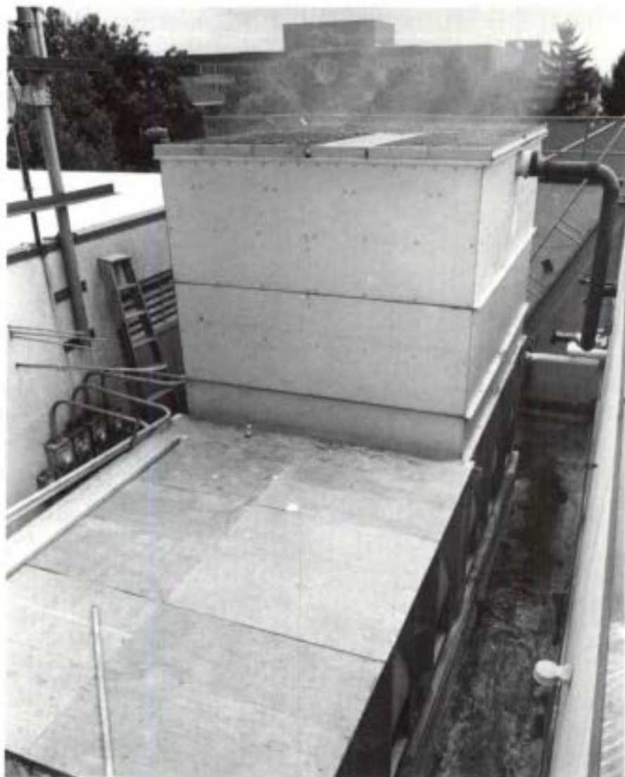
One of two "open" cooling towers.
