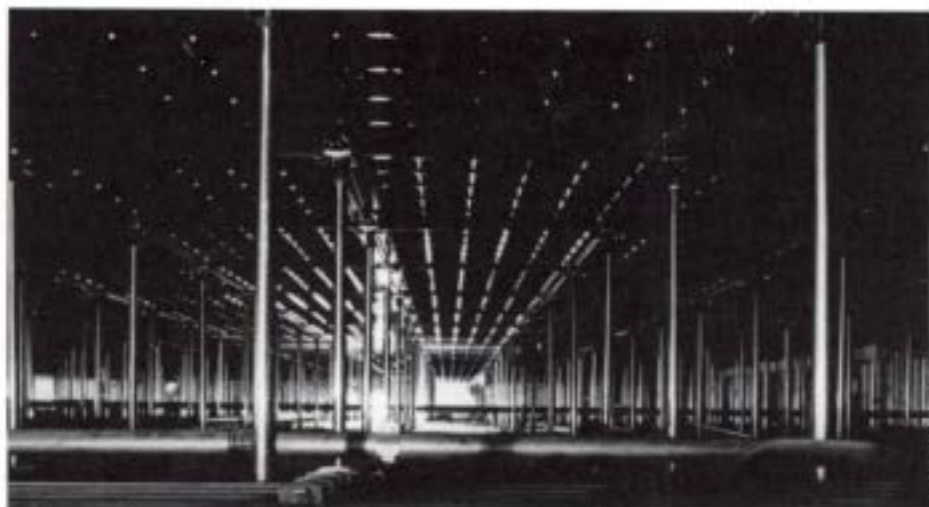
Lighting under computer floor for safety and maintenance.
