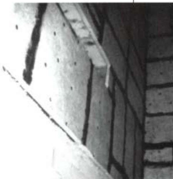
Moisture causing fungal growth between insulation panels due to moisture incursion.
