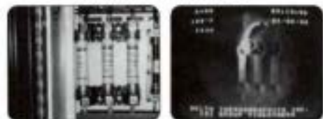
The infrared picture at right shows the cartridge fuse hot (white) and running at 188° F.
