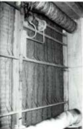
Roll-type pre-filter should be used before more efficient filters and should be changed on a regular basis. Roll is broken.
