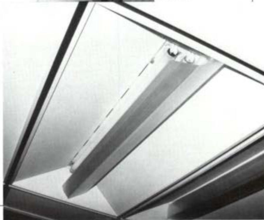
Poor air distribution around fluorescent lights and exhaust causes poor air movement.
