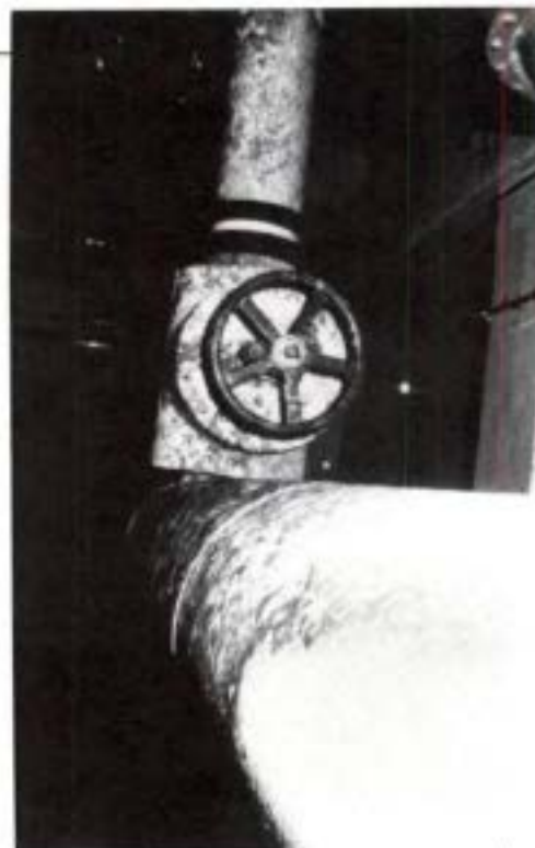
Microbial growth on pipe wrapping due to excessive moisture.
