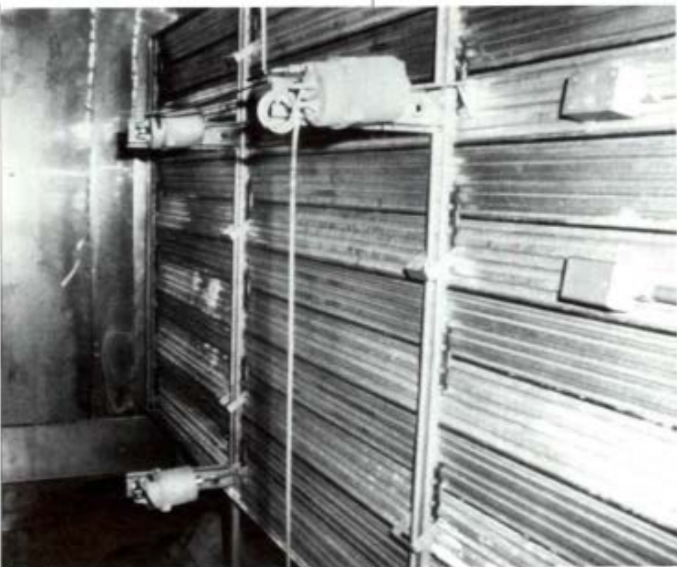
Fresh air intakes closed.
