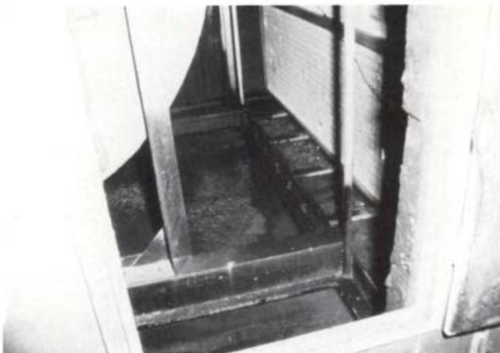
Standing water in air handling unit leads to microbial growth and dispersion of same.
