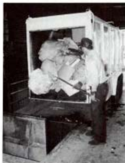
Loading refuse into incinerator hopper.
