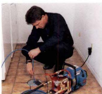
CLOGGED FLOOR DRAINS
