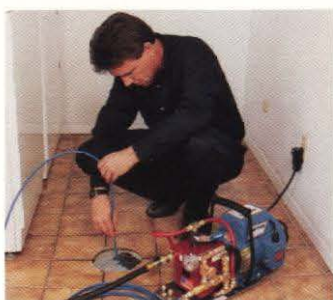
CLOGGED FLOOR DRAINS
