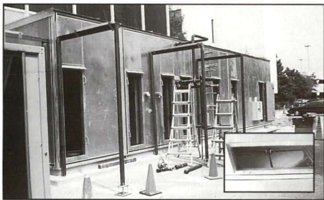
A desiccant cooling wheel and system outside the Medical College of Georgia's Research and Education Building.
