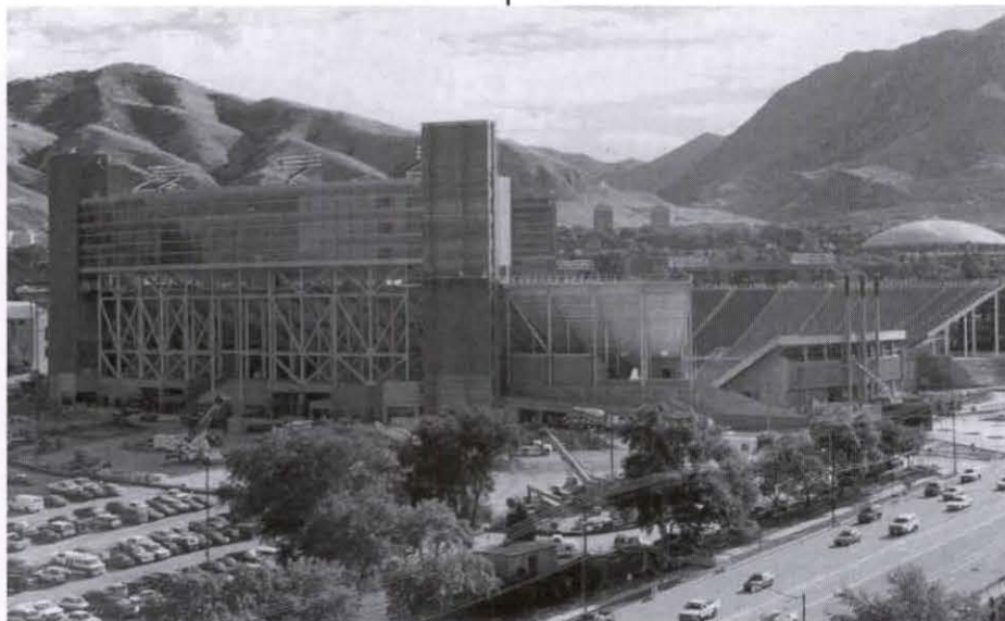
June 1998. Finishing touches are being applied to the bowl. Old scoreboard has just been removed. Stairs towers are growing sandstone skin.
