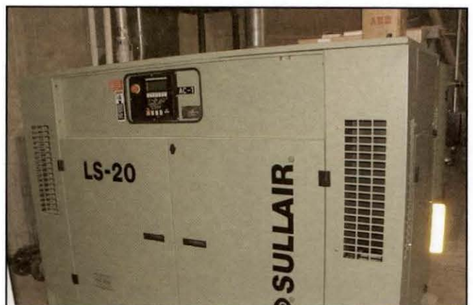
New main plant air compressor
