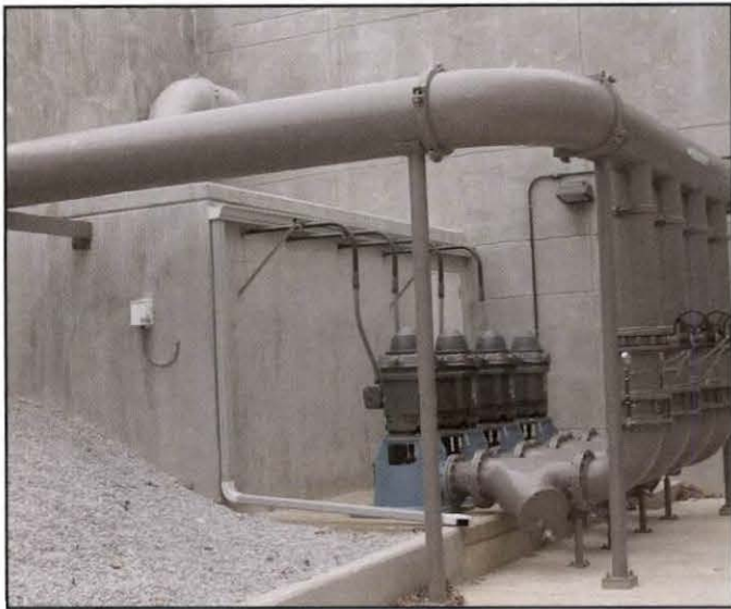
Southwest Chiller Plant condenser pumps
