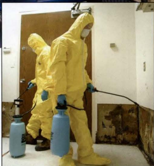
After Hurricane Charley, Munters restored St. Joseph's hospital in only two weeks. Services included cleaning, water removal, drying and mold remediation.
