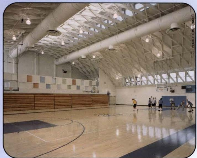
South Gymnasium with new clerestory glazing and ventilation system
