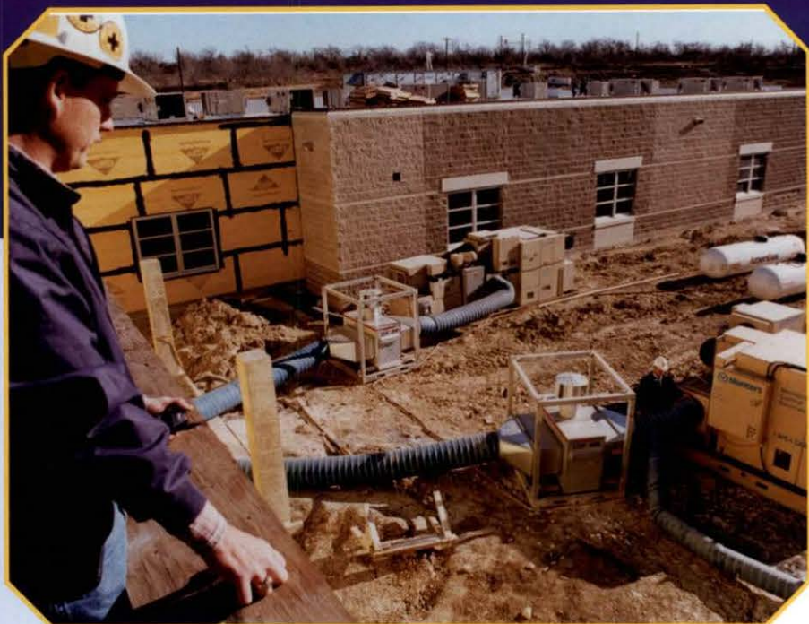
Desiccant dehumidification underway at an elementary school construction site near Austin, Texas.
