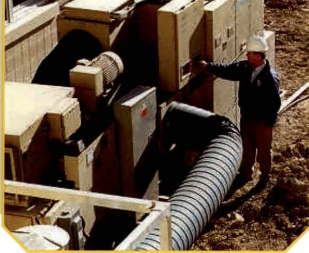
A mixture of desiccant dehumidifiers and indirect fired heaters is powered by a propane-fueled generator to operate the heaters and the blower fans, eliminating the need for an electrical connection.
