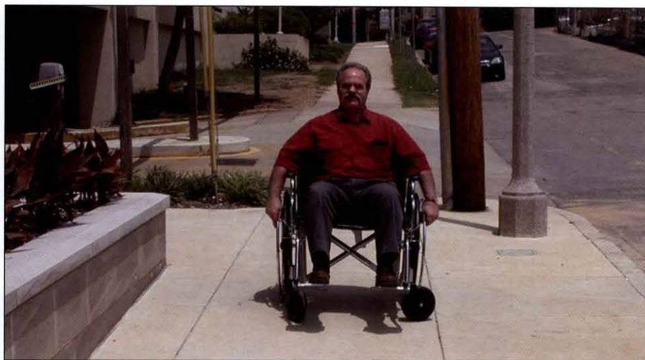
This cross slope is within the requirements of ADA.
