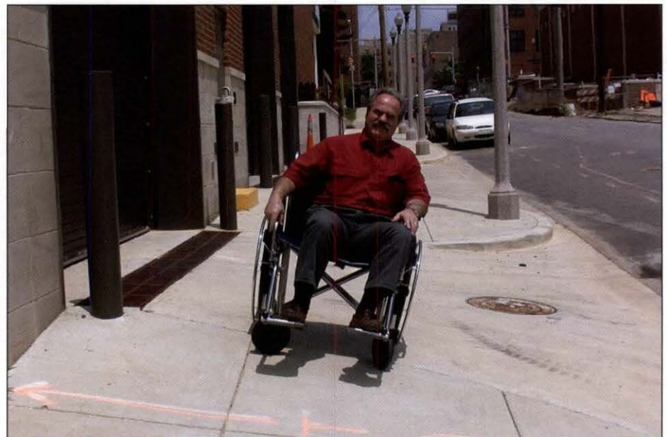
This cross slope is too steep and is an example of what happens when finish grades and spot elevations are not checked and confirmed by the design professional during construction.
