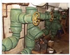
Pipe Fitting Components Insulated with Cut 'n Wrap
