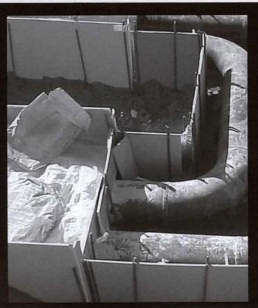
Gilsulate has insulated and protected underground pipes and tanks for over 60 years. This federally approved, patented system is economical, thermally efficient and hydrophobic. Gilsulate®500XR is load-bearing and provides a dry, stable environment for the long-term reliability of underground piping systems operating between 35° and 800° F. Examples of its many applications include steam, condensate, hot and chilled water.
