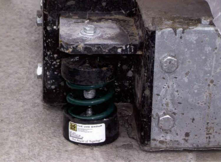
SPRING ISOLATOR SHORT CIRCUIT
