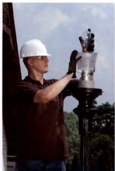
3. Remove Lamp and Refractor
