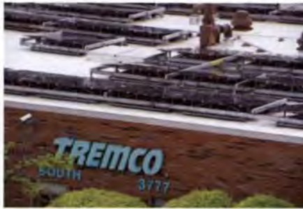
Photovoltaic Roofing System
