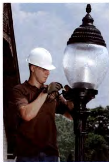
5. Connect Power to LED Conversion Kit
