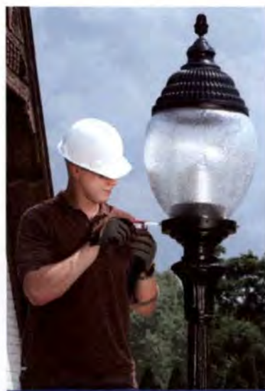
6. Tighten Set Screws
