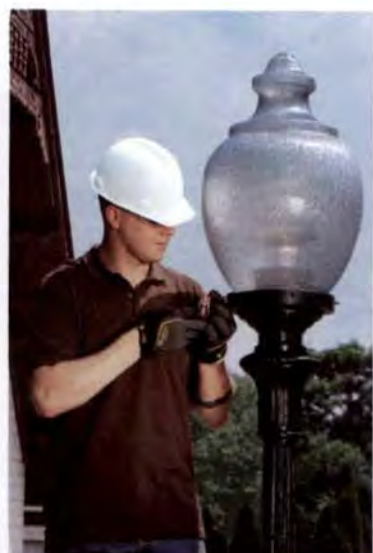
1. Loosen Set Screws
