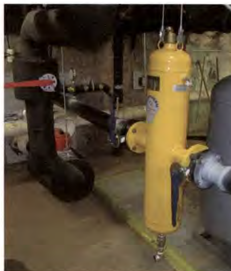
Spirovent Air / Dirt Separator Pummill Hall
