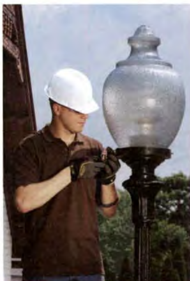
1. Loosen Set Screws
