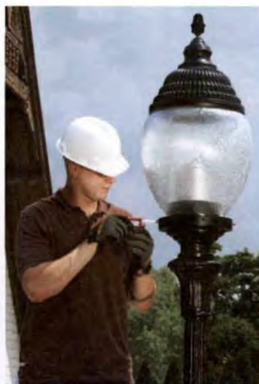
6. Tighten Set Screws
