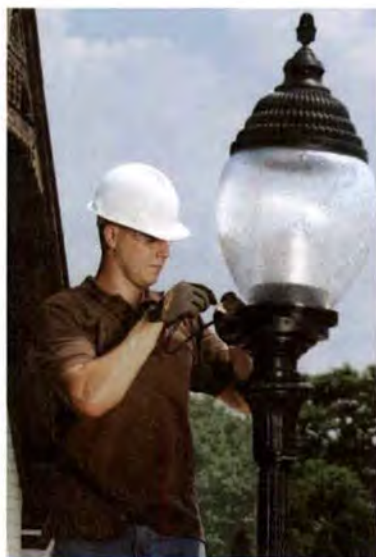
5. Connect Power to LED Conversion Kit
