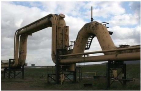
The photograph shows large industrial pipes with expansion joints, illustrating the practical application of expansion solutions in a real-world setting.
