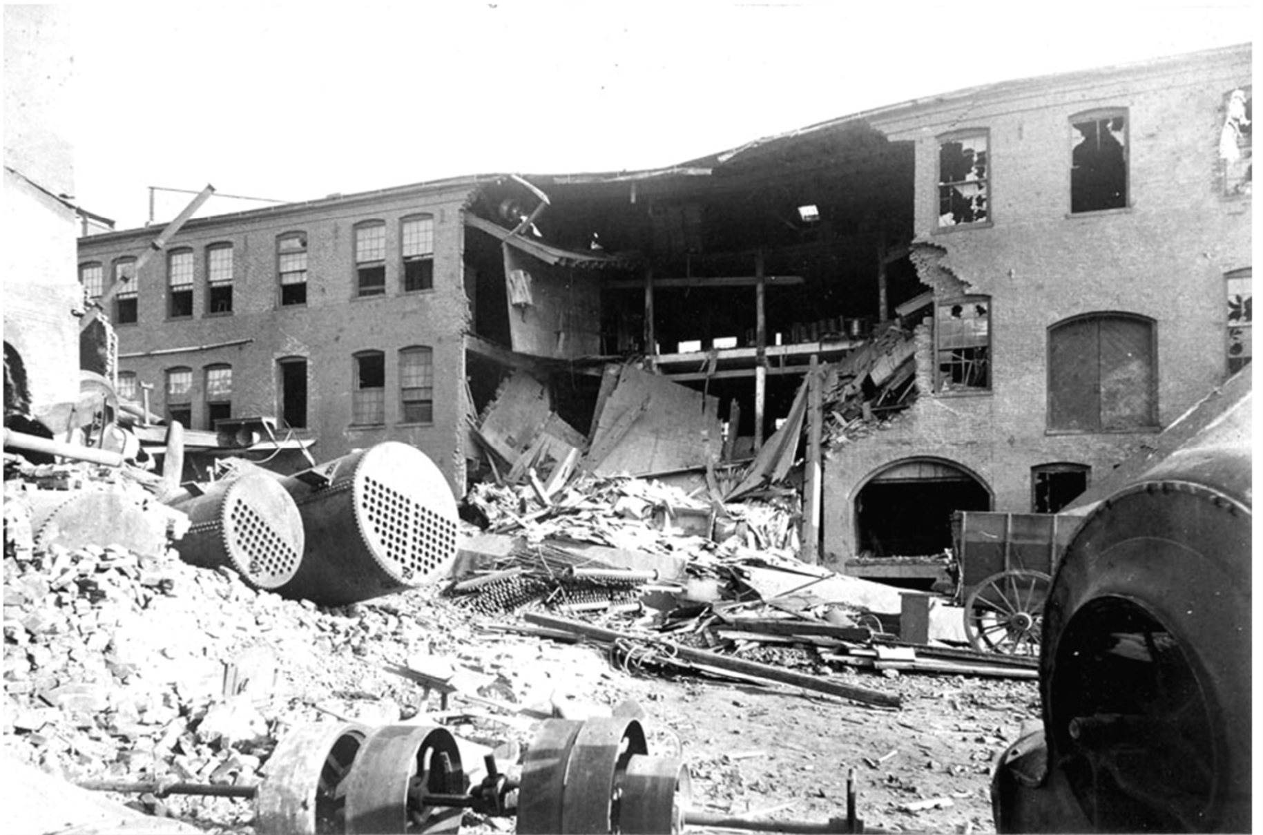
BOILER EXPLOSION AT BEAVER MILLS, KEENE, N. H., MAY 22, 1893.
